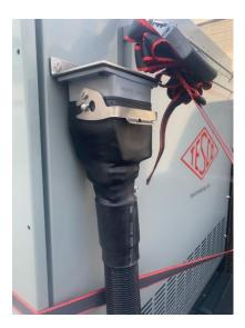
Ensure the breaker cover is secure and tight. This is for waterproofing.
