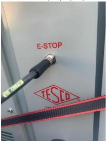
Before any transport, ensure the Staubli connector is properly secured to the L-bracket and the latch is down and tight so that it cannot move. This also ensures the connector is waterproof. The connector works by aligning the pins into the square and pushing the silver bracket down with force until it locks.
